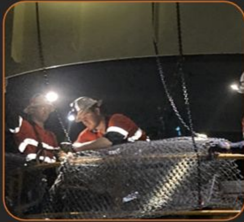
Installed scribing mesh
