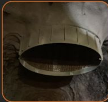
Created plug with 90 cubic meters of shotcrete
